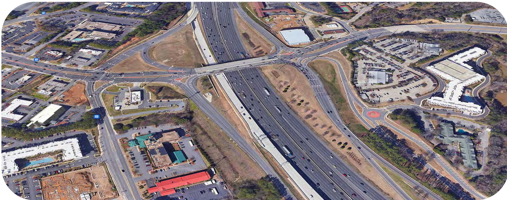
I-75/Windy Hill Road/Diverging Diamond Interchange, Cobb County, GA
